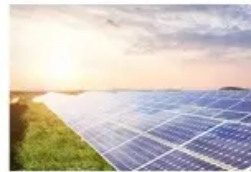
Energy Storage System
