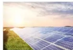
Energy Storage System
